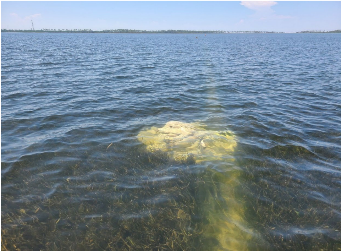
Figure 13. Sediment tubes staged adjacent to a propeller scar in preparation for installation.
