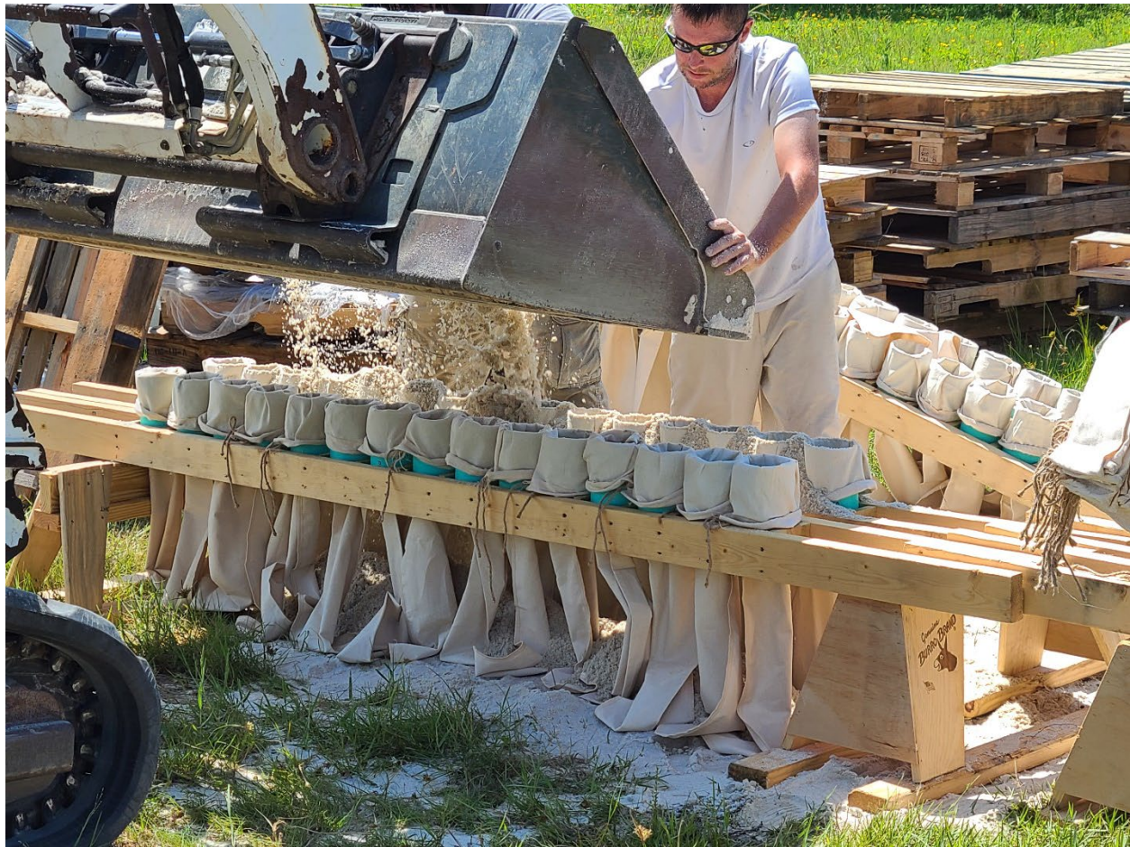
Figure 7. At the fill site, several sediment tubes were filled at a time using a skid steer loader.
