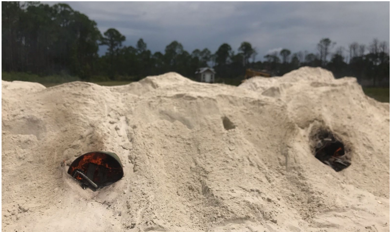
Figure 8. Fires were built within the sediment pile to keep it dry despite summertime storms
