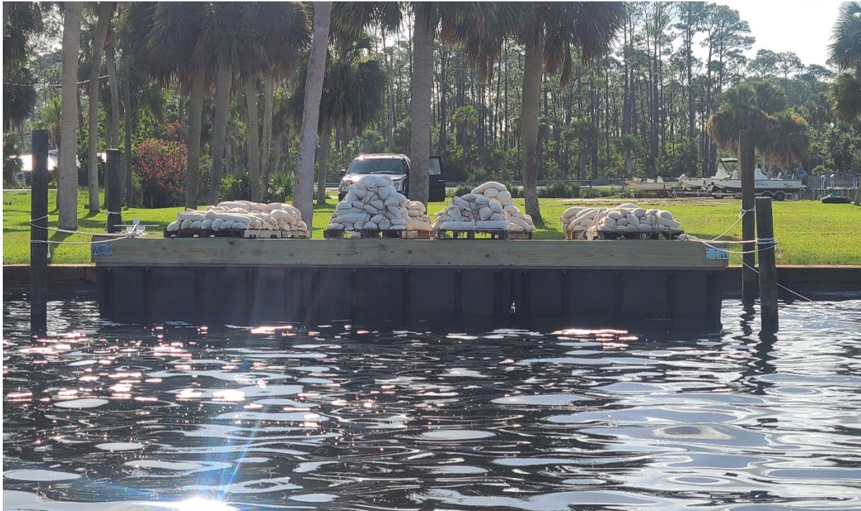
Figure 10. Filled sediment tubes on the floating platform staging area at Presnell's Marina, ready to be transported to the restoration area for installation.
