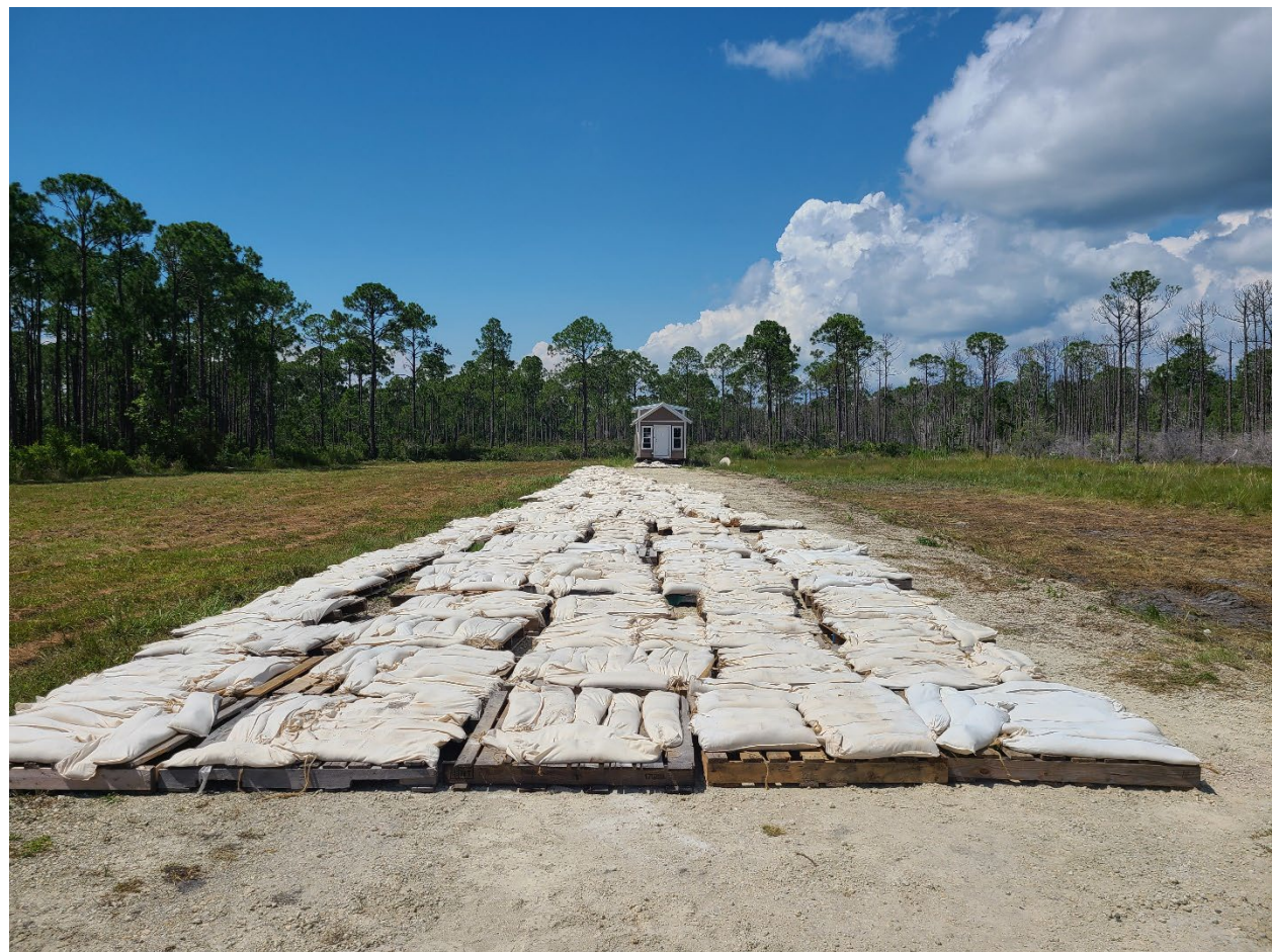
Figure 9. Filled sediment tubes laid out on wooden pallets, awaiting transport to the staging area
